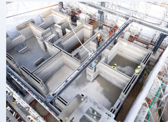
◆ 建筑3D打印 Architectural 3D printing
